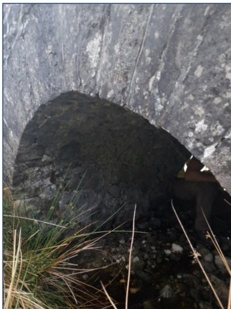
Plate 4-27 Stone arch Bridge 3 located near T5.
