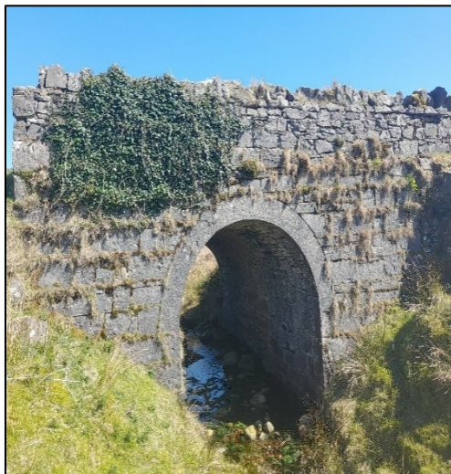
Plate 4-23 Bridge 1 – a stone arch bridge which is located near T6.
