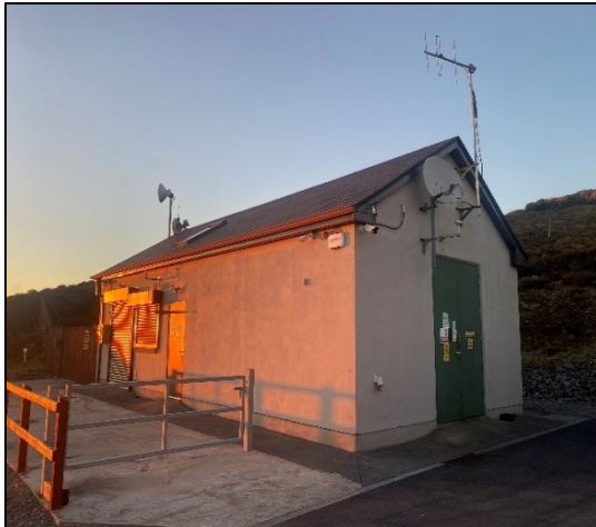
Plate 4-19 Exterior of Kingsmountain control building.
