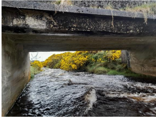
Plate 3-3 Example of a bridge structure within the Proposed Wind Farm site, showing limited structural features and assessed as having Negligible suitability for roosting bats.
