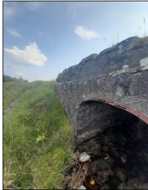
Plate 4-26 Face of Bridge 2 – stone arch bridge.
