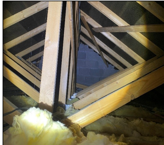
Plate 4-20 Attic space within the control building. No lighting present, torch used to illuminate photo.
