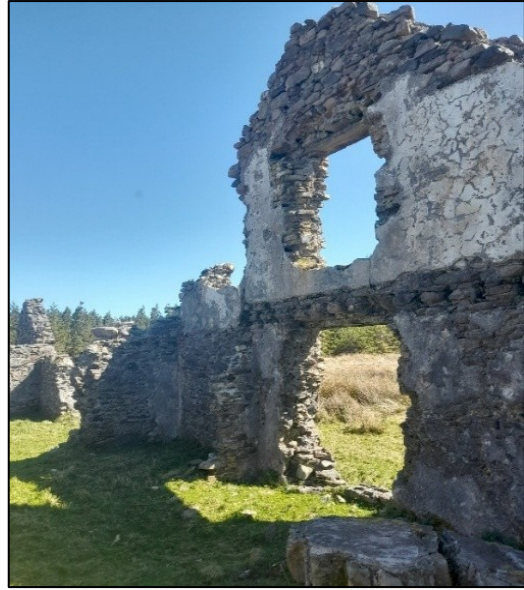
Plate 4-18 Second angle of Old stone ruin - gaps in stonework visible
